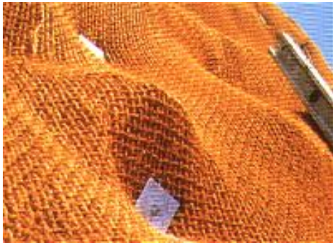
Fig.8 Secured by using wooden stakes as pictured here [4].
