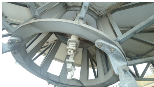
Figure 13.15 Feed Horns
