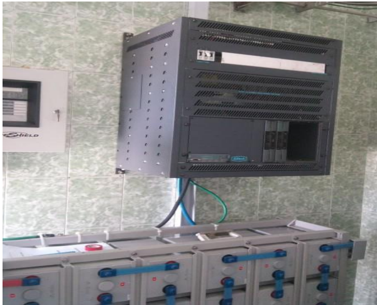
Figure 31: Rectifier which rectifies the AC Voltage into DC.
