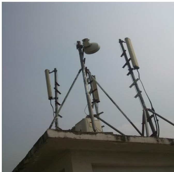
Figure 33: GSM microwave antenna
