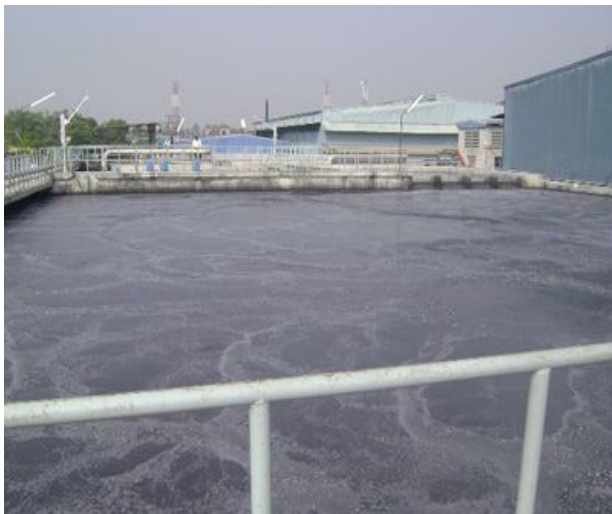
Biological Effluent treatment plant
